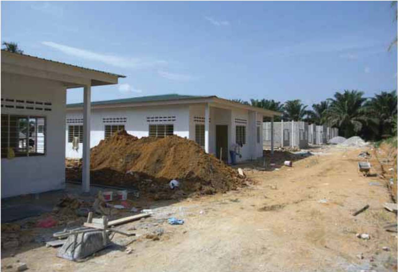
■ Construction of New Labour Lines - Buloh Akar Estate
