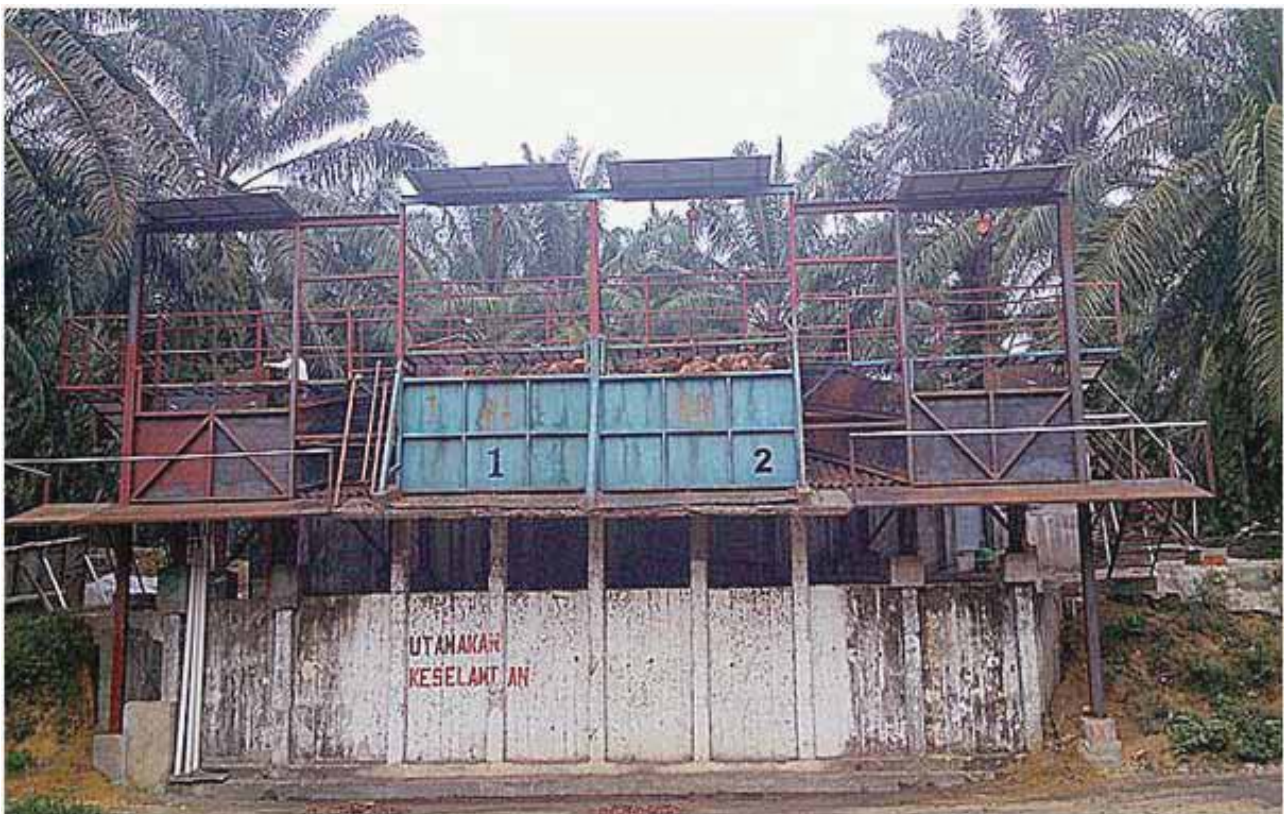
■ Ramps with Chain Block Doors - Narborough Estate
