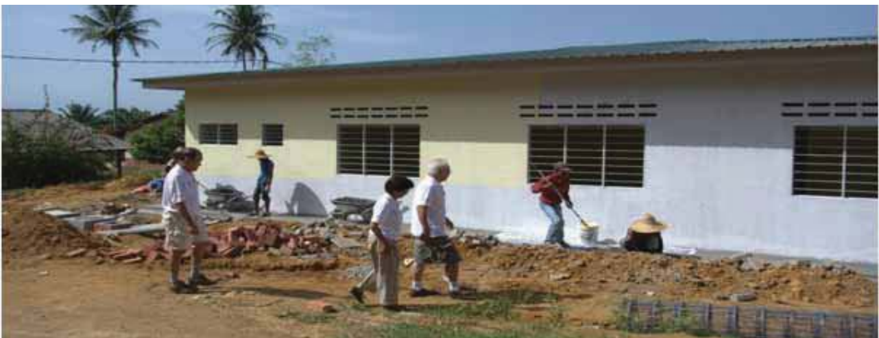
■ Construction of New Labour Lines - Narborough Estate
